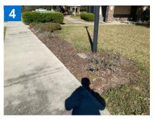
1 Near playground area bank along sidewalk is eroding leaving a drop-off and exposing irrigation piping. Recommend adding soil and Bahia sod to eliminate potential trip hazard.
